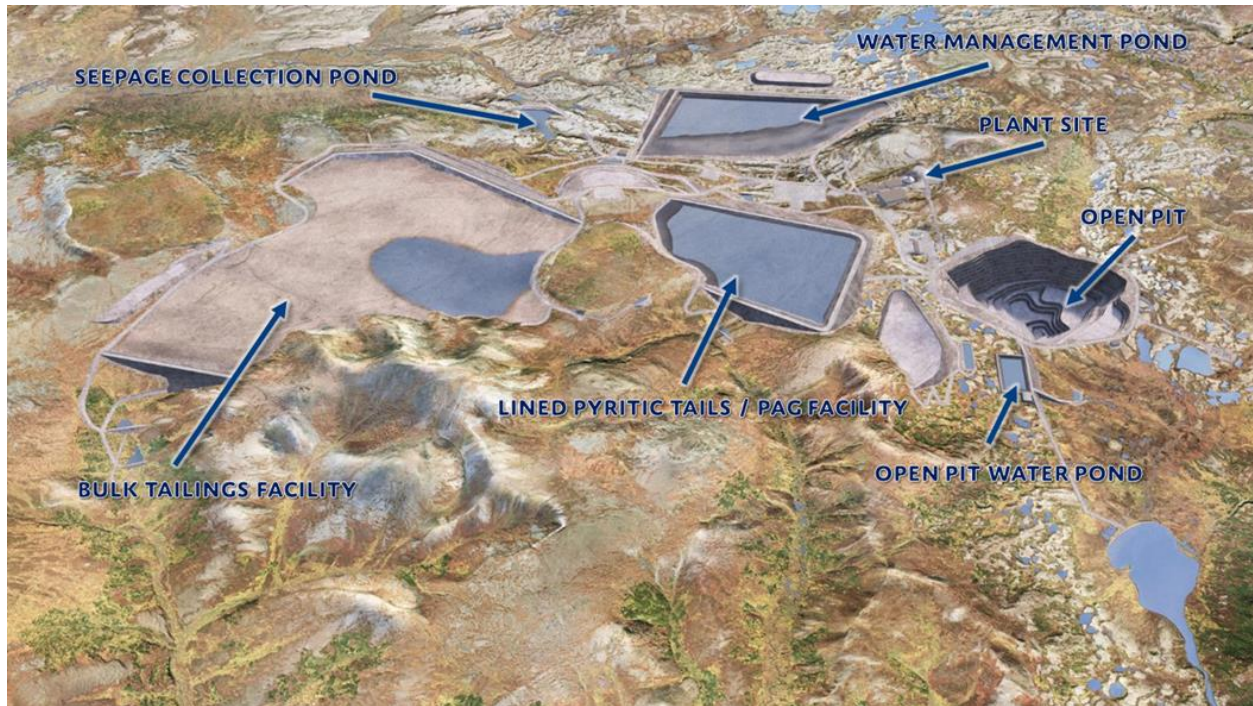
Figure 2 illustrates how proposed mine-site facilities have been grouped closely together, reducing the overall footprint of the mine and providing other environmental benefits, such as reduced energy use in water pumping.
